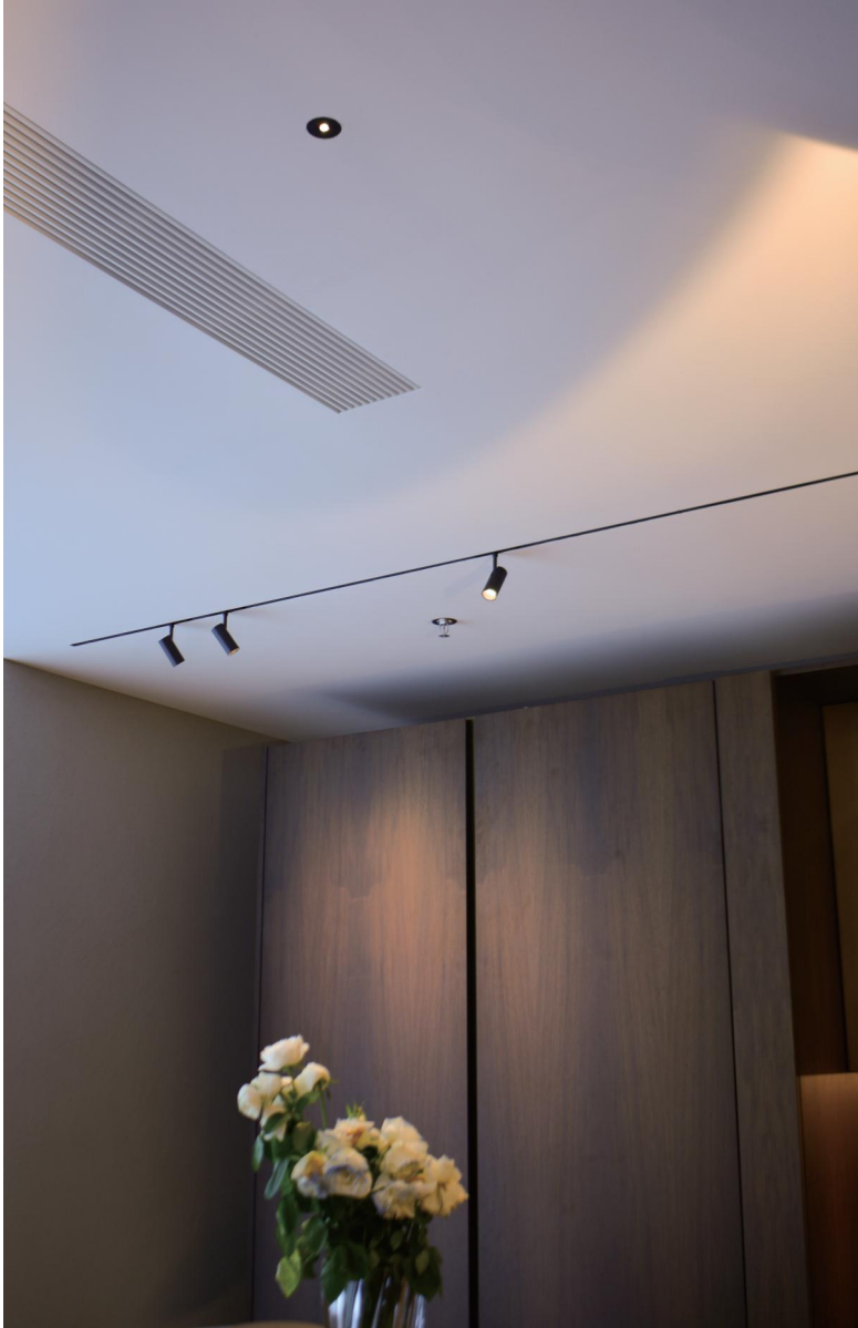
DuraGreen project: Rimadesio Showroom
